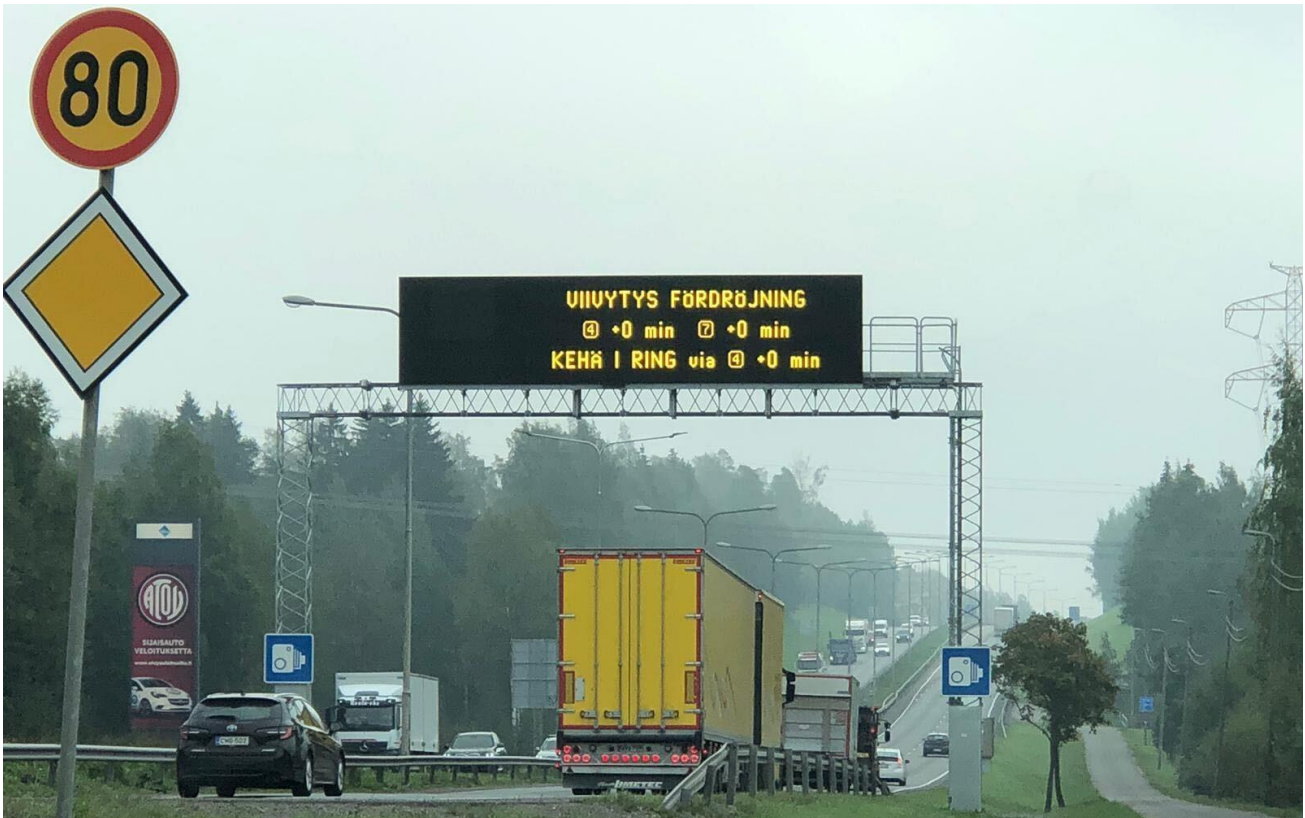
Figure – Presentation of travel time delays derived from Waze’s travel time data in the VMSs on Ring Road III.
